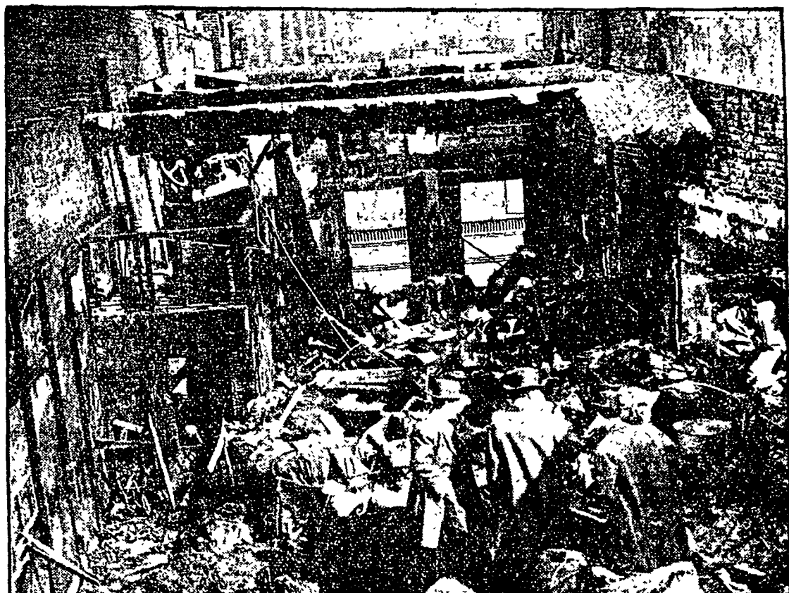
LOOKING DOWN THROUGH THE ROOF OF 40 AND 42 SUMMER ST AFTER THE FIRE.
