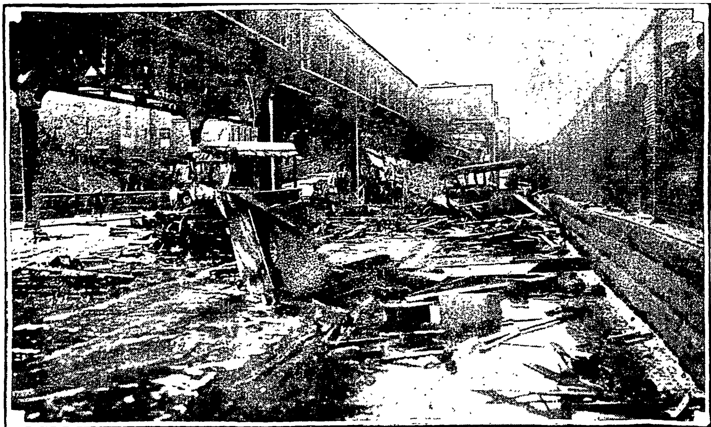
A VIEW ON COMMERCIAL ST.
